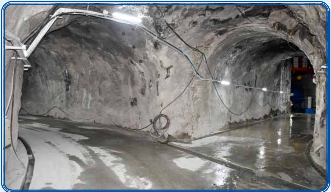
Adit-2 & Valve Chamber Bifurcation
