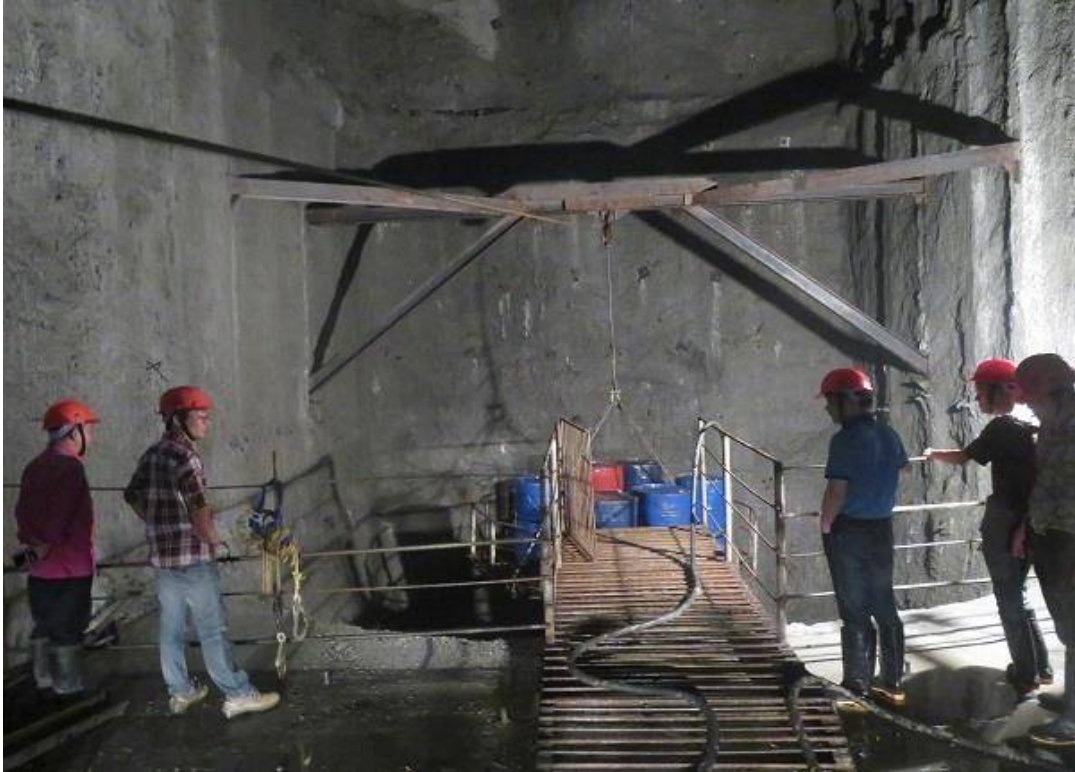
Support Frame at Vertical Shaft
