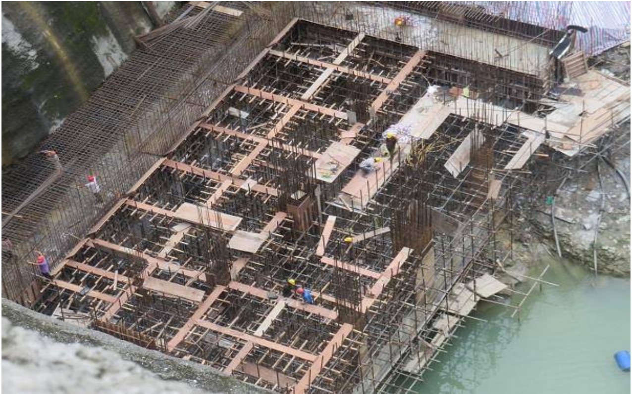
Auxiliary Power House Construction
