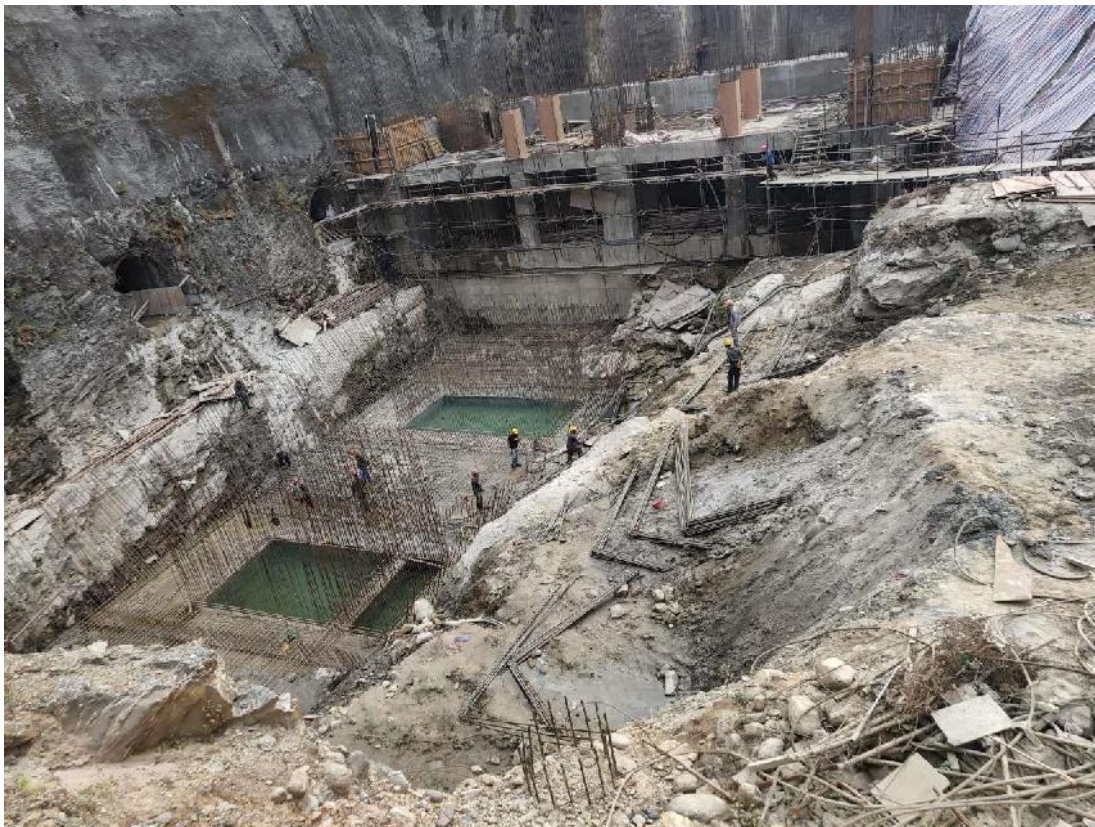
Construction of Machine Hall
