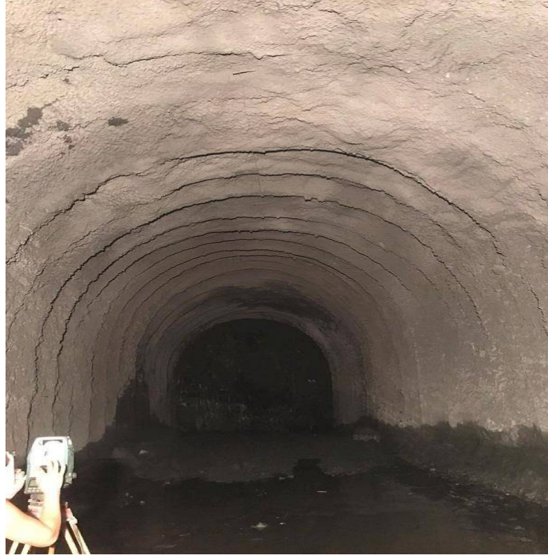
Excavation and Support of HRT
