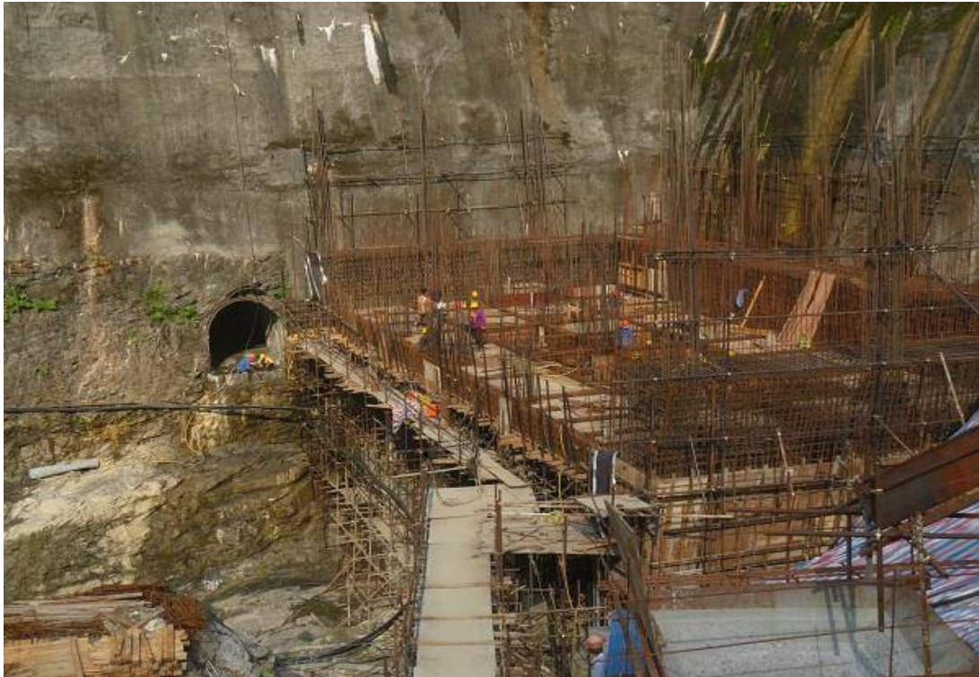
Auxiliary Power House Construction
