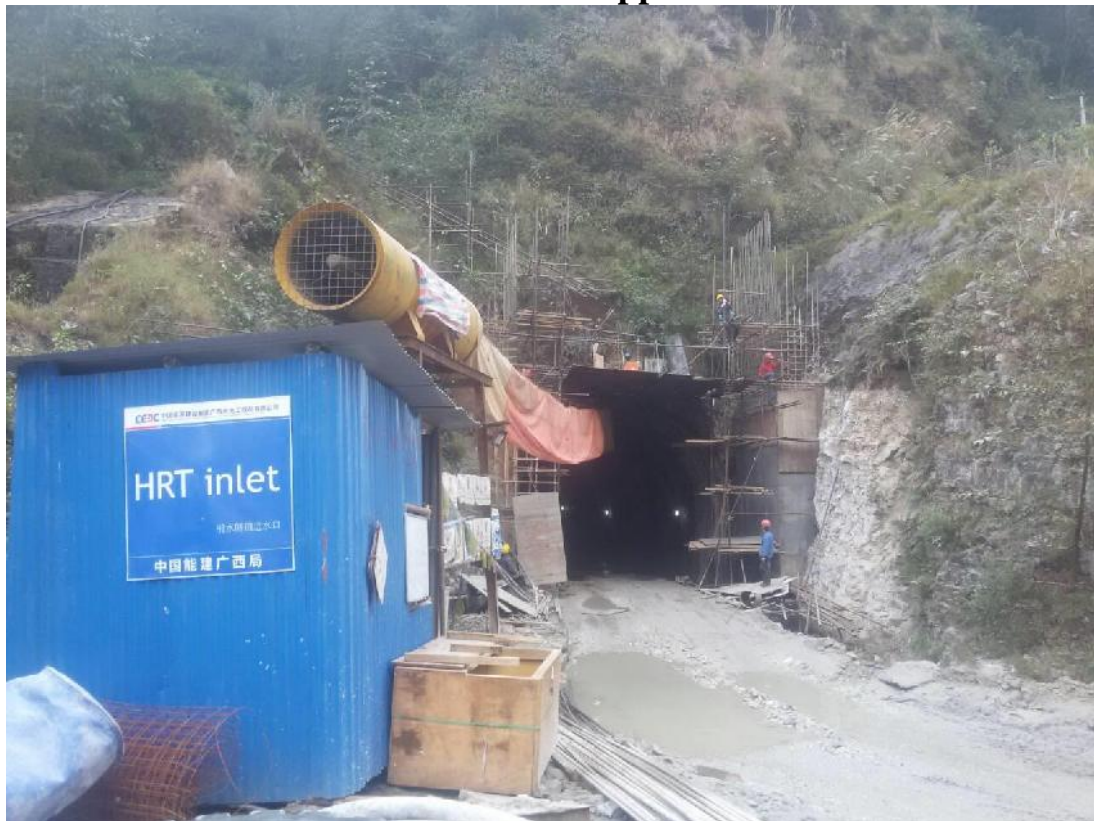
HRT Inlet Tunnel at Chaku
